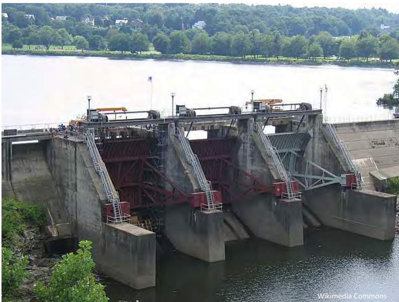
Figure 1. FirstLight Power dam in Turners Falls MA.
